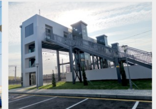
▲ Location: Azerbaijan Project Name: Railway station 24-21
