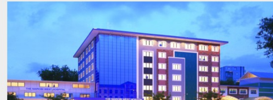
▲ Location: Kenya Project Name: West Hospital Nairobi
