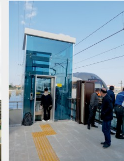
▲ Location: Azerbaijan Project Name: Railway station 24-1
