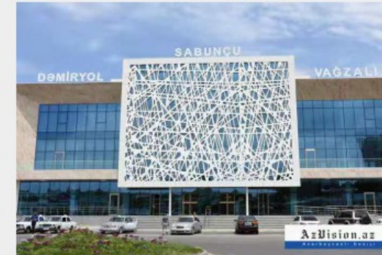
▲ Location: Azerbaijan Project Name: Railway station 24-15
