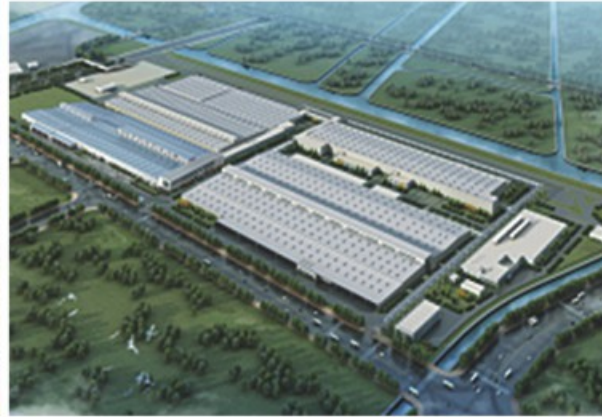
▲ iland factories Myanmar 12 units Cargo lifts
