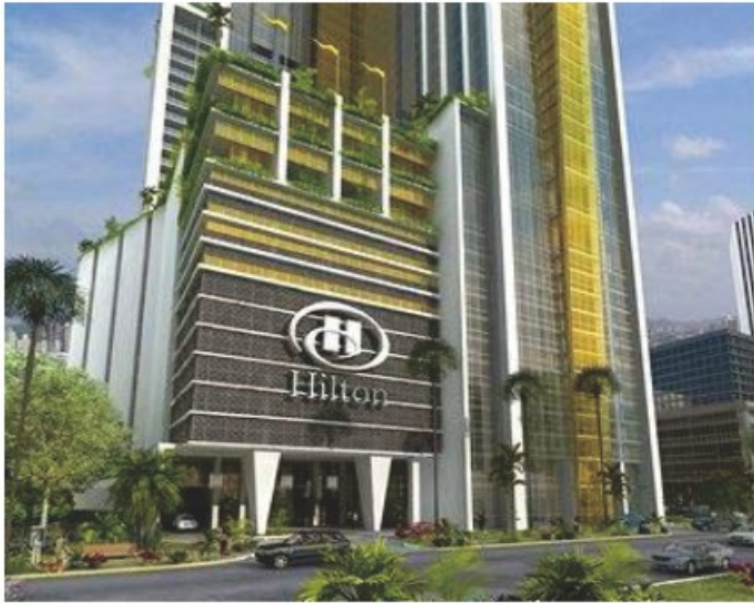
▲ Location: Panama Project Name: Hilton Hotel
