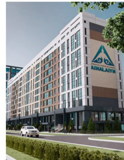
Location: Kazakhstan Project Name: Astana Sani
